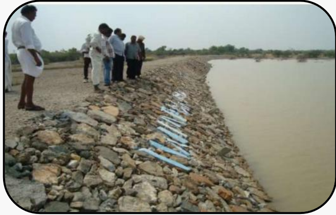
Surface Technique-Percolation Tank
