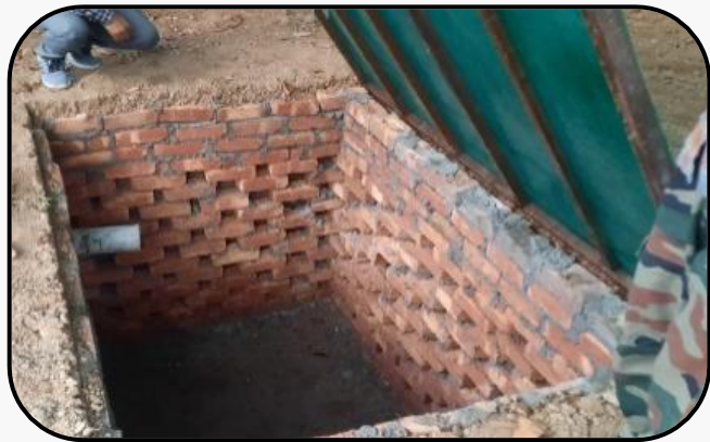
Sub-Surface Technique: Recharge Pit
