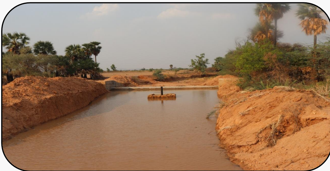
Percolation tank with Recharge shaft
