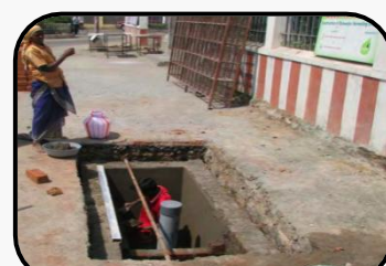
Trench with Borewell
