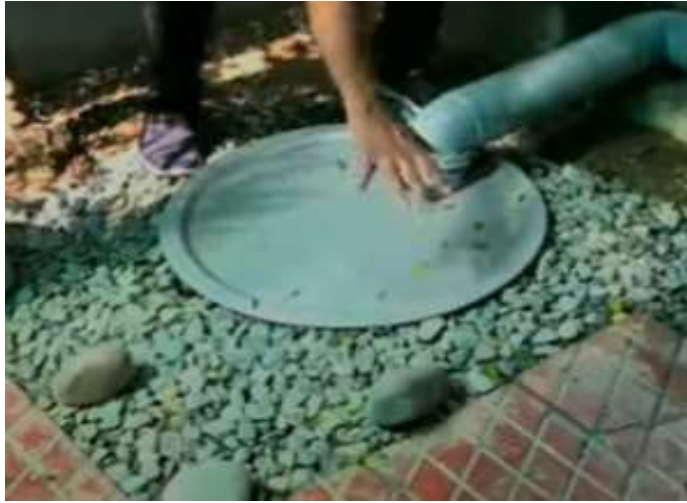
07) Gravel Filling at Periphery and inside entire pit and covering it from top with lid
