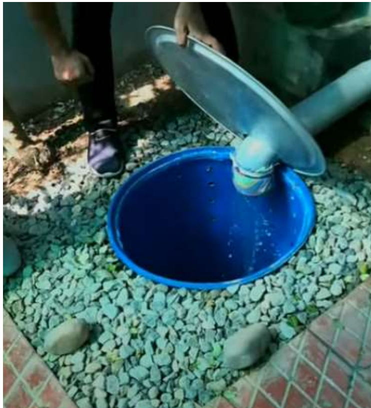
07) Gravel Filling at Periphery and inside entire pit and covering it from top with lid
