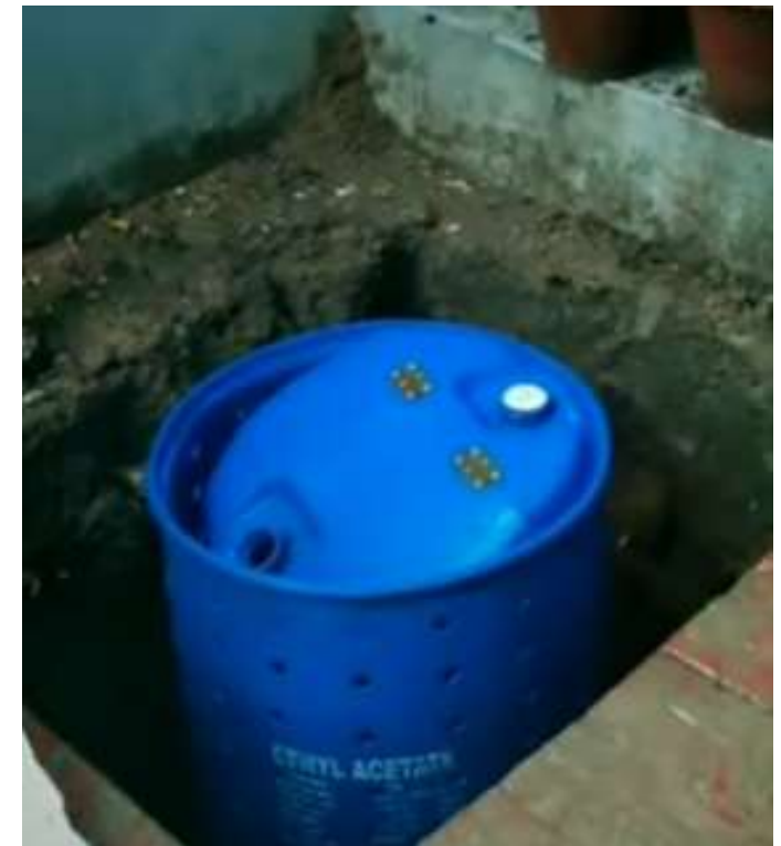
06) Barrel Positioning inside pit
