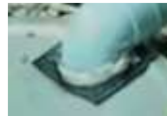
06) Jali to avoid penetration of dust particles
