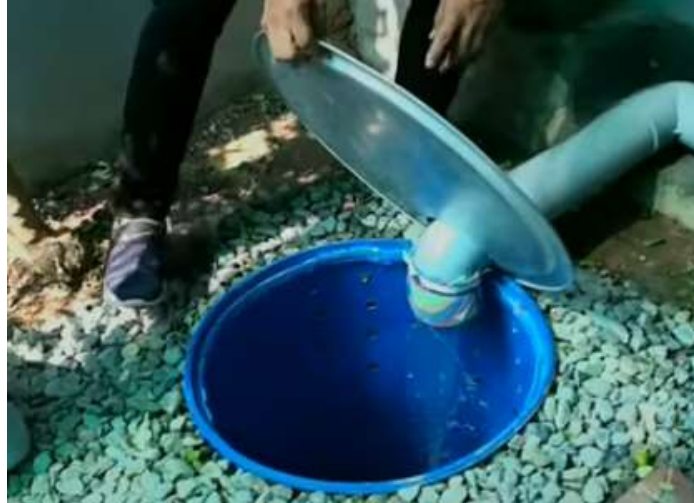
08) Covering Pipe with Cloth for filtration from pebbles or rocks
